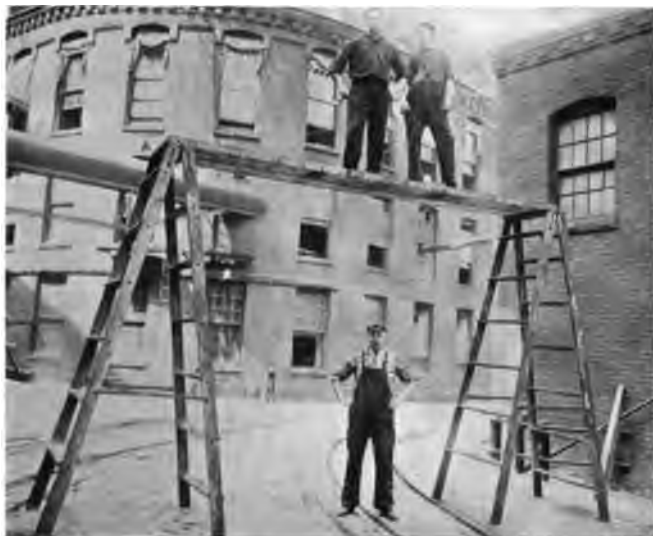
Fig. 2. Staging, set up.*
